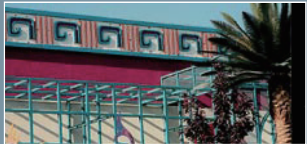
Panel Cresting on Casino • 51 1/2" Height • 68" Length of Panels
