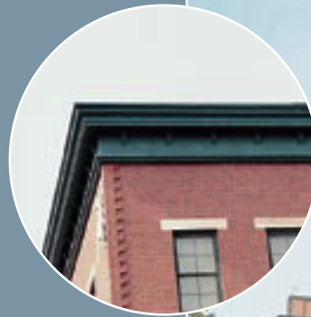
Moulding with brackets, pre-finished in the factory
